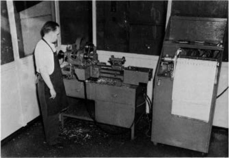
The Arma lathe, with punched-paper control unit. One of the earliest N/C machines. Courtesy of Frederick Cunningham, Jr.
